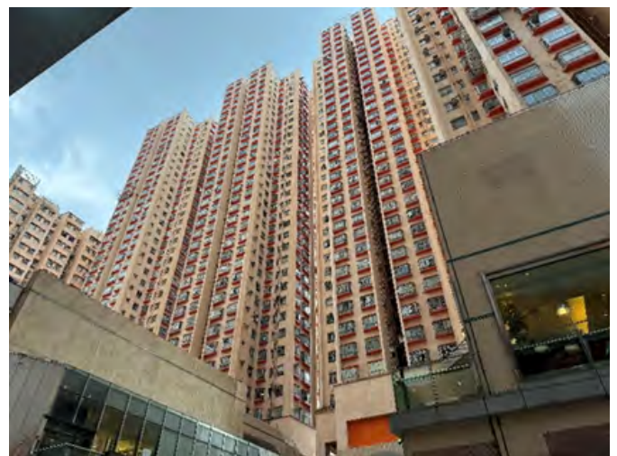
A variety of restaurants and shops are provided at the arcade beneath Amoy Gardens.
