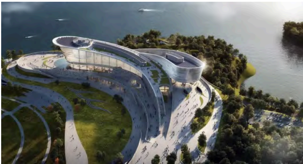
Rendering of Science Museum located at North Riverside Park, Wanzhou District, Chongqing City. (Source of Photo: Wanzhou District Government)
